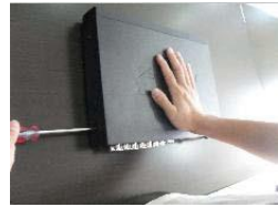
⑥ install the screws on both sides of shell
